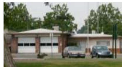
Rio Linda Fire Station showing original brickwork
