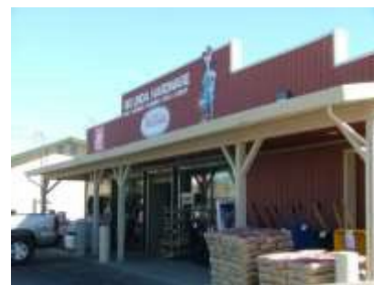
A typical commercial building, with flat roof and false front, wood siding, and an awning
