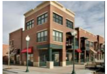
The third story incorporated into the corner of this mixed-use building allows for additional square footage without compromising the building's human scale. Varied setbacks and rooflines provide visual texture and articulation.
