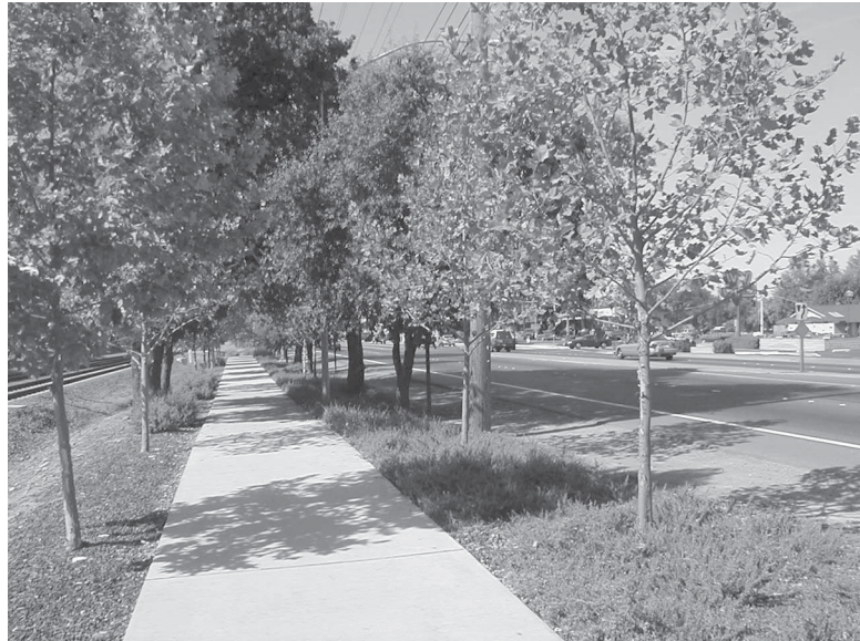
Separated sidewalk along Folsom Boulevard, just west of the Mather Field/Mills LRT Station.
