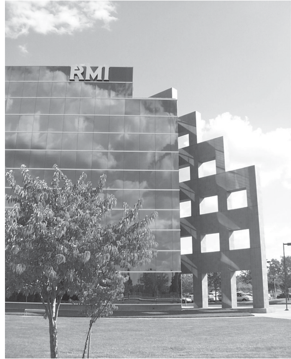
The RMI building located within the Capital Business Center south of US Highway 50.
