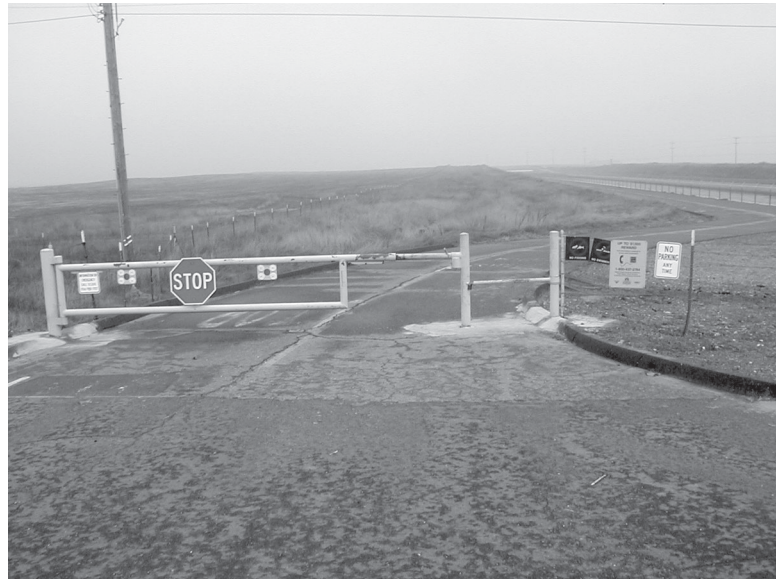
Gated entry to the Folsom South Canal bicycle trail at Jackson Road.
