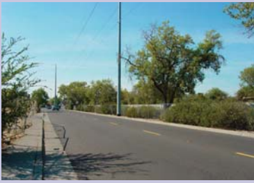
Existing sidewalk locations hinders pedestrian safety
