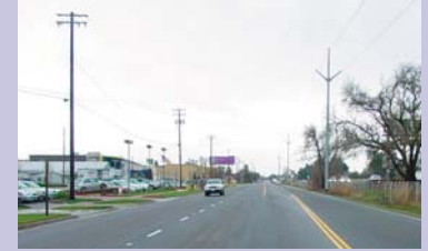
Power lines detract from the Boulevard's appearance
