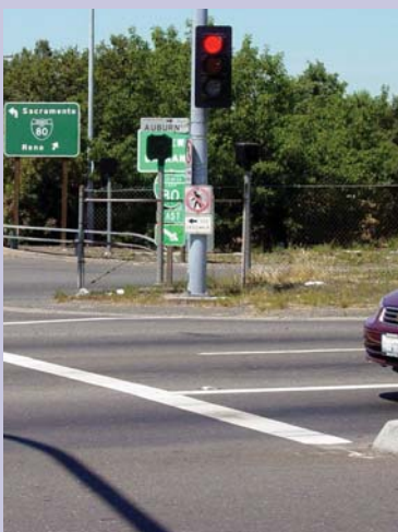
Poor crosswalk configurations limit pedestrian access to and from West Auburn Boulevard
