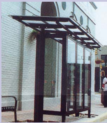
Bus stop shelters are oriented to face adjacent properties instead of the street
