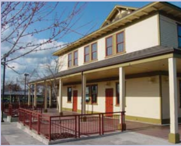
The Mills Station in Rancho Cordova is an example of how an historic structure can be preserved and reused to make a positive contribution to the character of Auburn Boulevard
