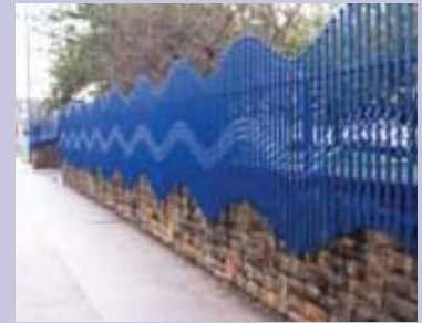
Approved decorative fencing and K-rail can enhance the Boulevard and contribute to traffic safety
