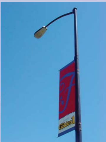
Street lighting will provide a safer atmosphere along Auburn Boulevard and create a unifying element
