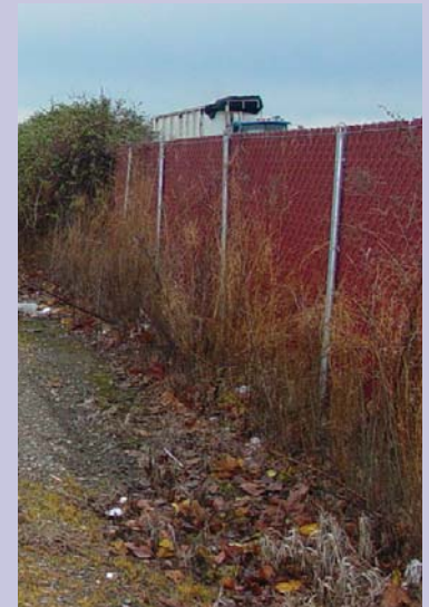
An unsightly Caltrans fence hinders views of the Boulevard from the Capital City Freeway
