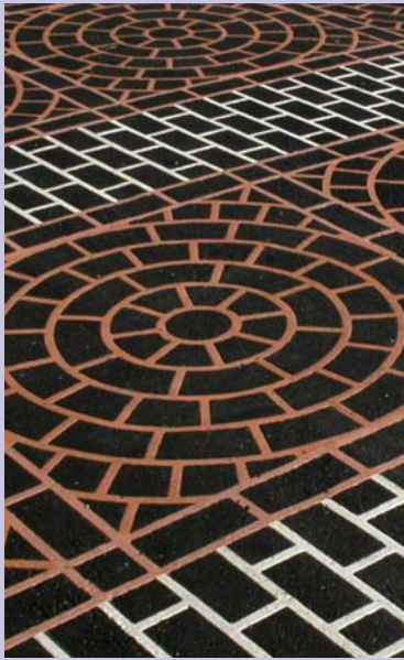
Duratherm decorative pavement will be used as an at-grade median where necessary, further unifying the character of West Auburn Boulevard
