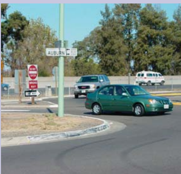
Current off-ramps from the Capital City Freeway disrupt traffic flow along West Auburn Boulevard
