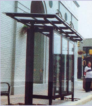
Bus stop shelters are oriented to face adjacent properties
