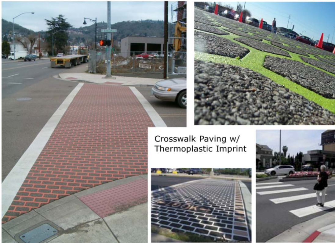
Figure 24 Examples of crosswalk paving with thermoplastic imprint
